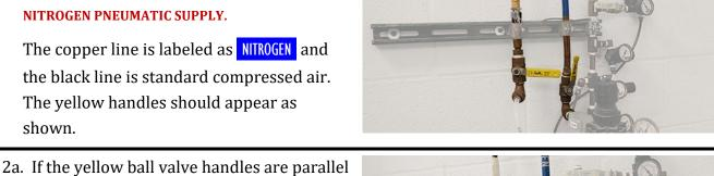
2a. If the yellow ball valve handles are parallel to the supply line, that line is open. If perpendicular, the supply is closed. If the instrument is still on the compressed air supply, the handles will be positioned as shown.
