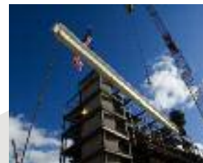
The signed beam is hoisted in place.
