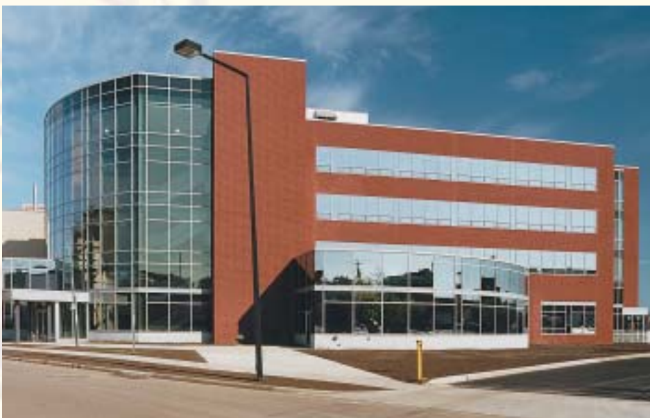
The Polymer Engineering Academic Center, above and at right, which is nearing completion, will be open for tours at the June 8 dedication ceremony.
