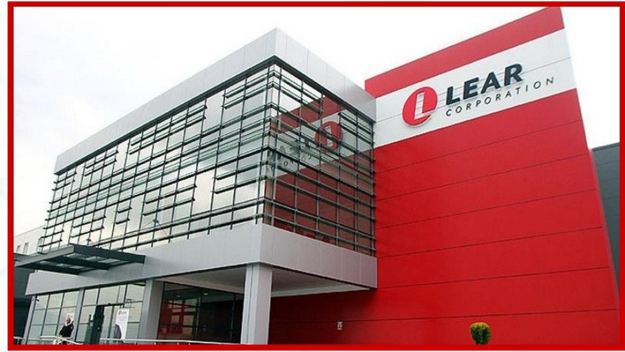
08.11.2016 - LEAR CORPORATION OPENED THEIR NEW PLANT IN THE TETOVO FREE ZONE
