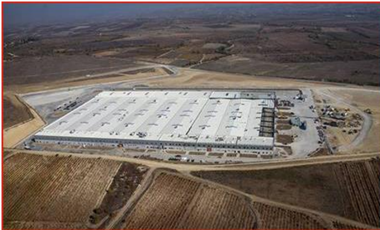
A MAJOR CLIENT FOR THE NEW FACTORY IN KAVADARCI IS MERCEDES-BENZ
