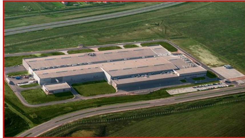
THE PRODUCTION FACILITY IN MACEDONIA HAS BEEN THE COMPANY'S LARGEST STRATEGIC INVESTMENT OUTSIDE BELGIUM
